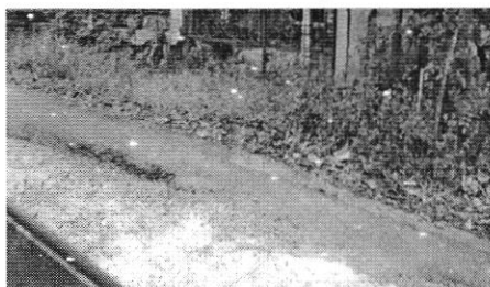
Figure 2 Road sinking due to lands under it landslides.
